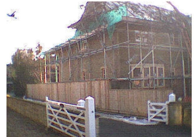
The frontal view (right) shows the "Bradstone" wall cladding is virtually completed on a dull, wet day and everything almost ready for the stone roof slates to be laid - whilst the view below shows the same elevation just a few days later with the stonework and roofing completed and the scaffolding gone!
